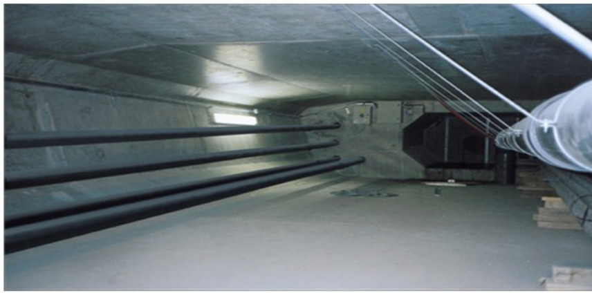
Figure 1.1: External Post-Tensioning in a bridge ( www.cclint.com )
