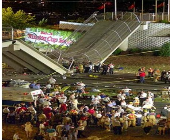
Figure 1. 7: Lowe's Motor Speedway Bridge Collapse, May 2000, US ( www.onlineathens.com )
